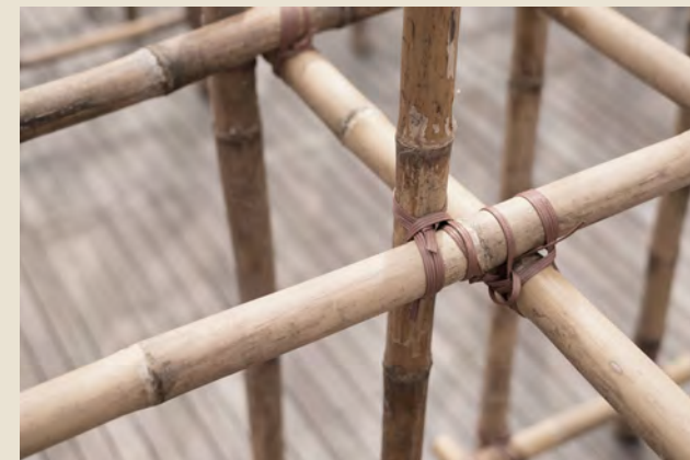
fig. 5 bamboo lashing
