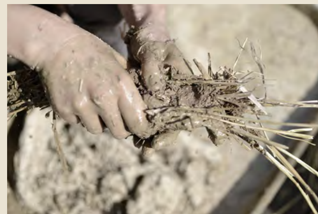
fig. 3 mixing COB
