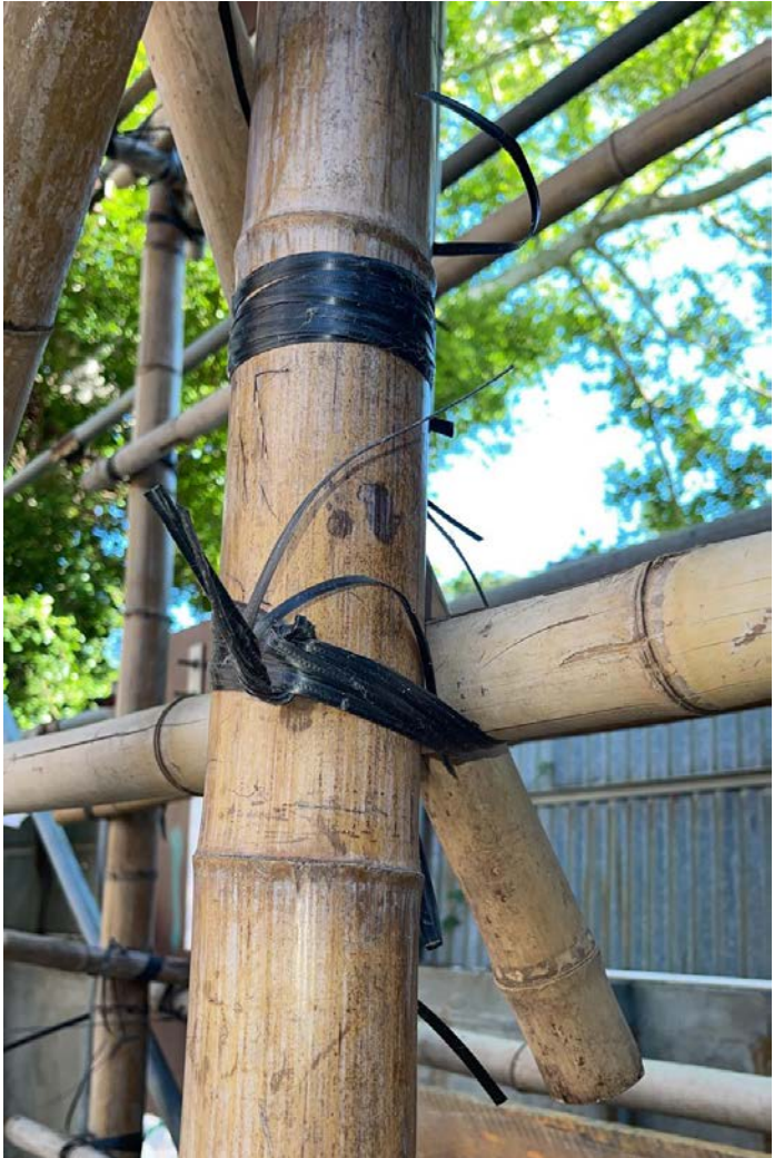
fig.19 Bamboo Scaffolding joints method (HKFTU Study Centre, 2021)
