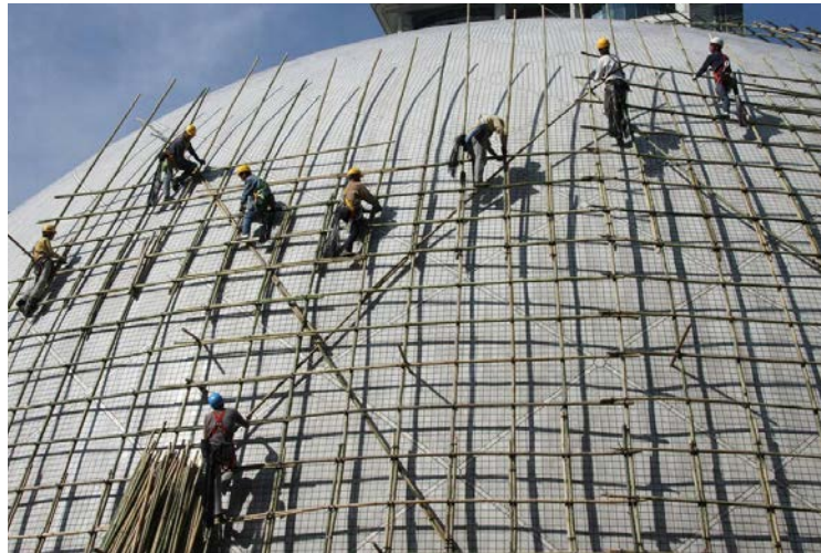
fig.18 Bamboo Scaffolding for building repairment (hkulifestyle, 2014)
